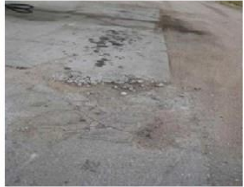
Excessive cracks
